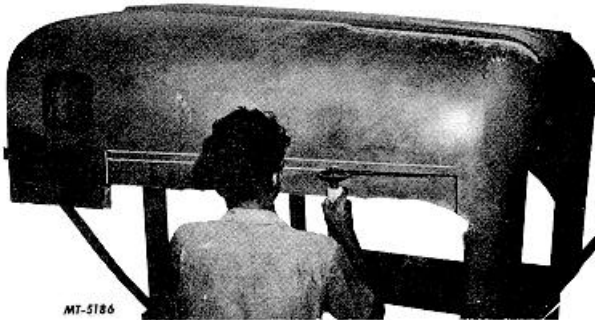
Fig. 8 Service Fender Cutout.
